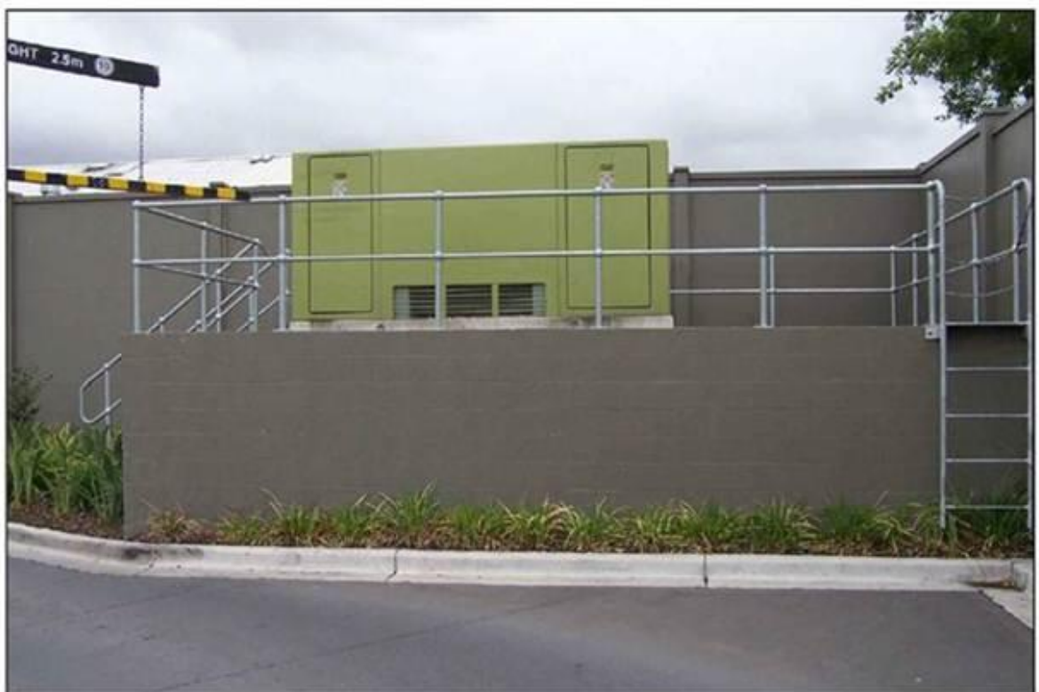
Figure 51 - Example substation raised above 1:100 flood level
